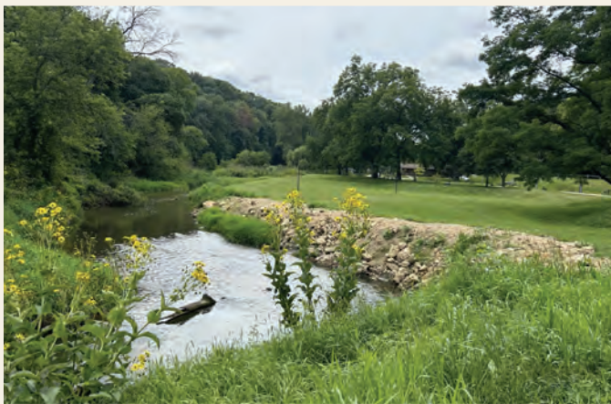
Bear Creek, which runs through Eden Valley Refuge, was ripped to prevent the bank from eroding into the campground.
