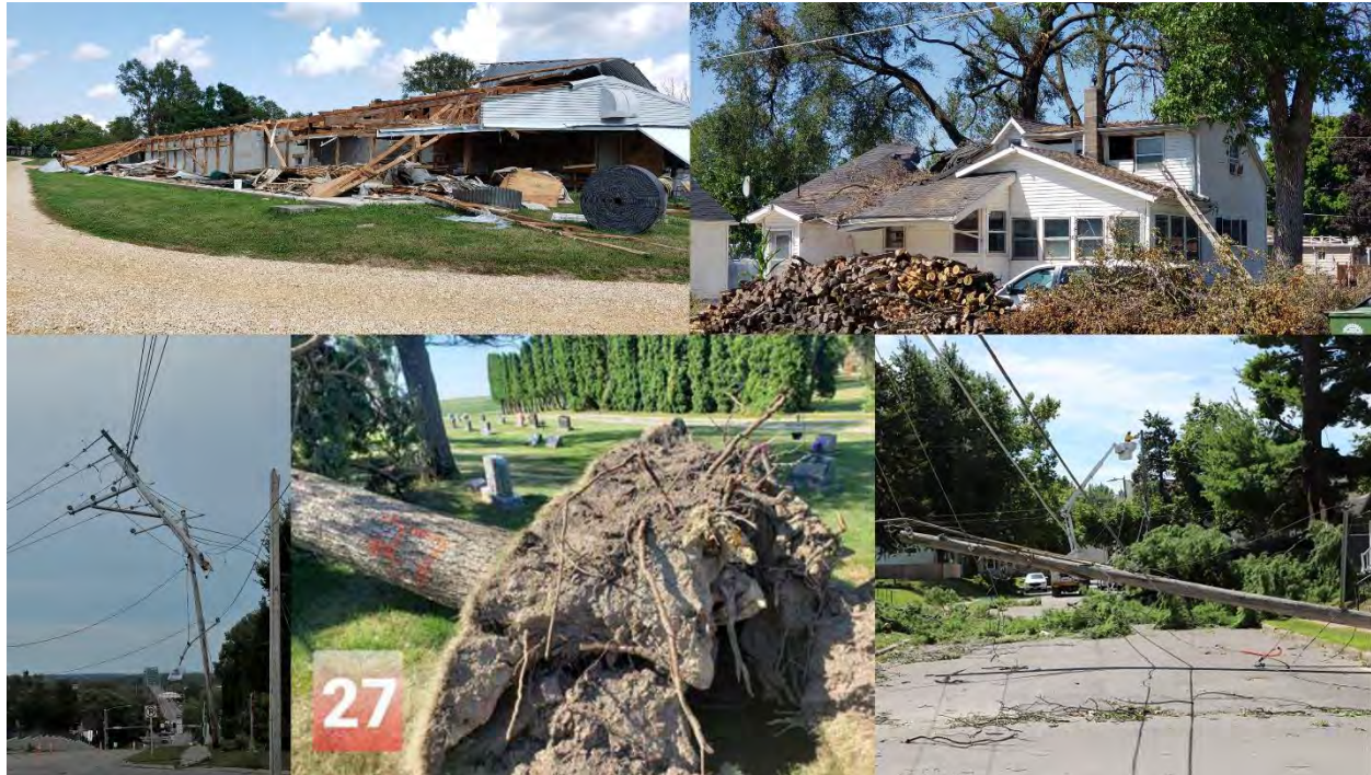
Figure 3-73 August 10, 2020, Derecho Damage
